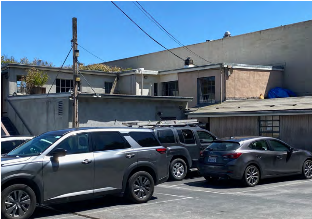
Figure 29: 605 & 607 Bridgeway, north and west elevations, "Auto" shed on right, looking southeast from parking lot (Turnbull May 2024)
