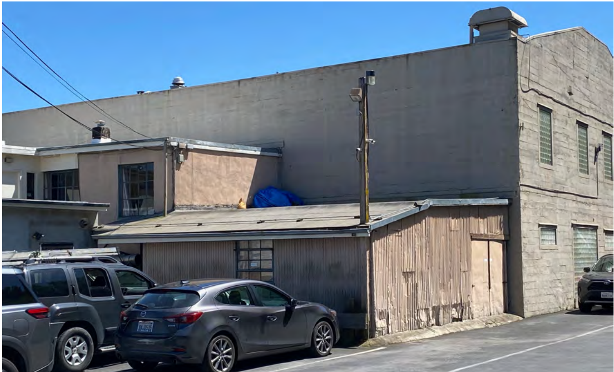
Figure 30: 605 Bridgeway, "Auto" shed (Turnbull May 2024)
