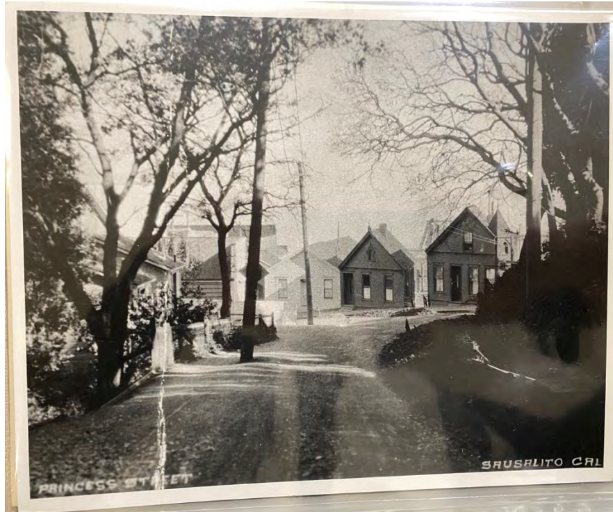
Princess Street dwellings, dark buildings are on lots J-K-L (Sausalito Historical Society collection, Edwin Long binder)
