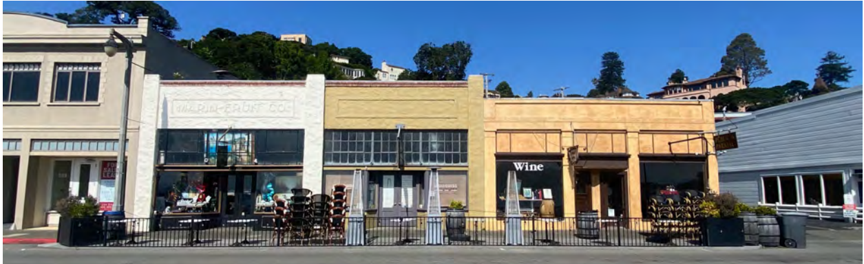
Figure 22: 605 & 607 Bridgeway and 611-613 Bridgeway (Turnbull May 2024)
