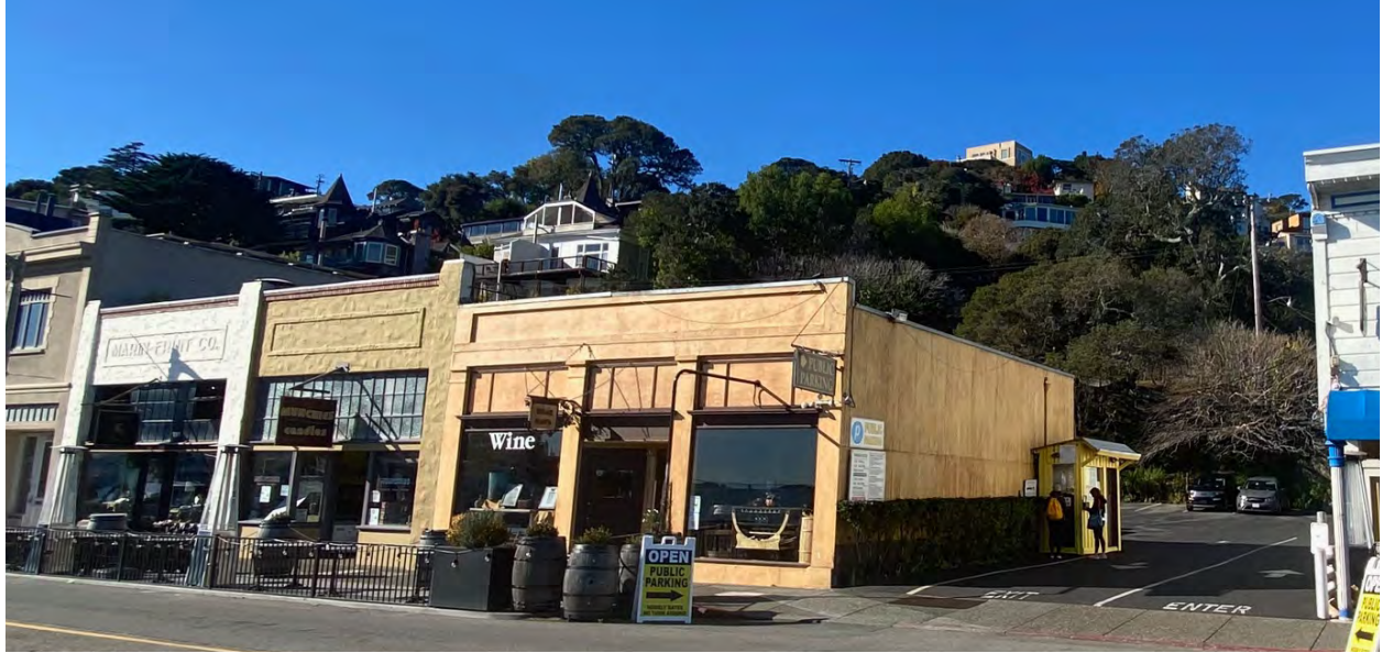
Figure 20: 605 & 607 Bridgeway on left, 611-613 Bridgeway on right (Turnbull May 2024)
