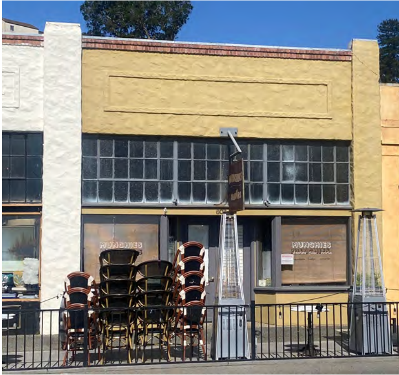
Figure 24: 607 Bridgeway, former Hong Lee Laundry (Turnbull May 2024)
