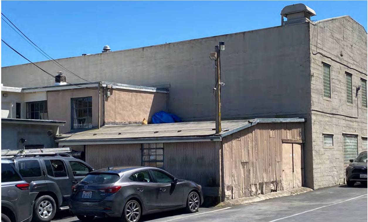
Figure 30: 605 Bridgeway, "Auto" shed (Turnbull May 2024)
