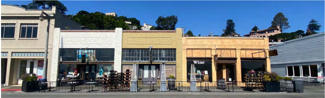
Figure 22: 605 & 607 Bridgeway and 611-613 Bridgeway (Turnbull May 2024)
