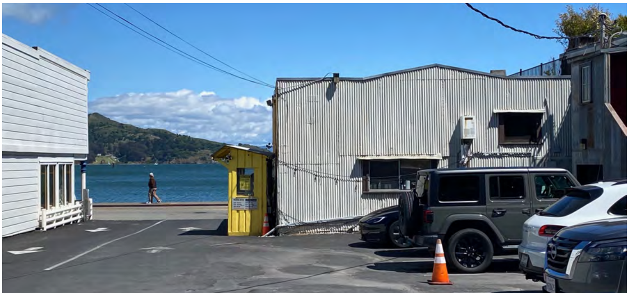
Figure 31: 611-613 Bridgeway, west elevations, looking east from parking lot (Turnbull May 2024)
